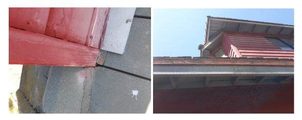
Rotten wood, leaks, improper installation:
