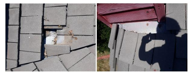
Improper flashing, no drip edge, tiles not past fascia:
